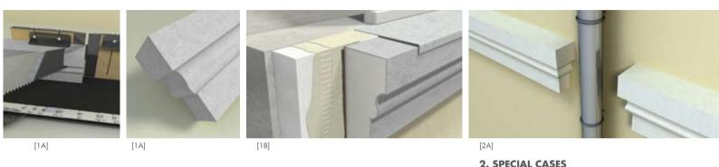
**[1A]** The ends of the window sills must be finished with corners cut at  $45^{\circ}$  (mitre cuts). To save time, the ends (corners cut at  $45^{\circ}$ ) can be assembled with the window sill before fastening to the façade (the day before, for example) or if not, at the same time as the installation.
