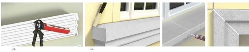
**[5B]** Then continue to lay down lines of adhesive over the entire surface to be glued (lengthwise on the moulding), spaced at +/-3 cm intervals.
