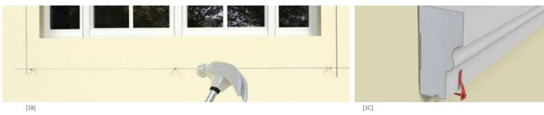
**[3B]** Drive the nails into the concrete on the lower line in order to hold the moulding in place (3 nails per length of 2 m). The nails will be pulled out after 24 hours.
