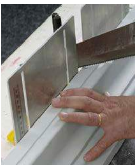
WINDOW SILL PROFILE ANGLED ON BOTH SIDES
