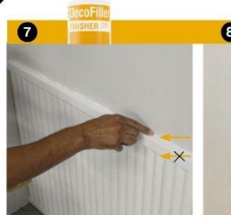
Use Filler to smooth out the visible joints and all vertical seams.
