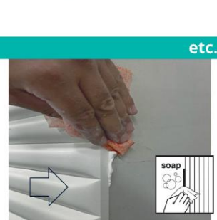
Push firmly and remove excess glue
