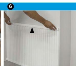
Push firmly and remove excess glue
