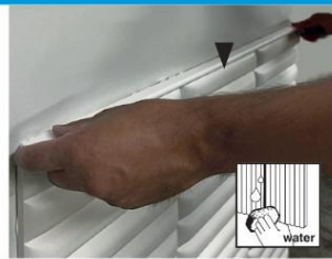
Apply Fix Power all around and on the length of the middle rib
