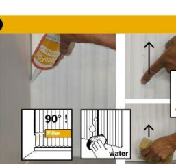
Use Filler to smooth out the visible joints and all vertical seams.
