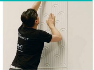
If desired, place a row of panels above the intermediate profile
