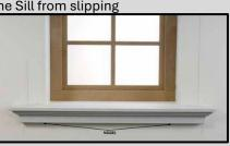
12. If required, install the functional External Window Sill, ensuring a proper slope for water runoff (see note above).
